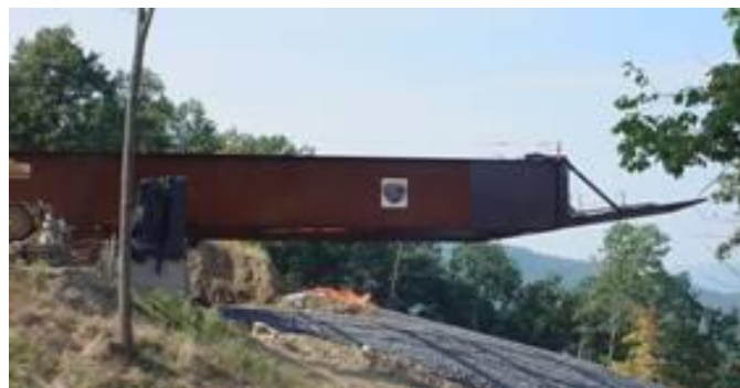
Figure 11 Photograph showing an I-girder bridge launching
