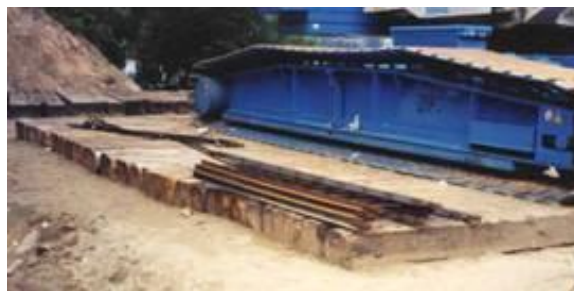
Figure 6 Photograph of a timber crane mat
