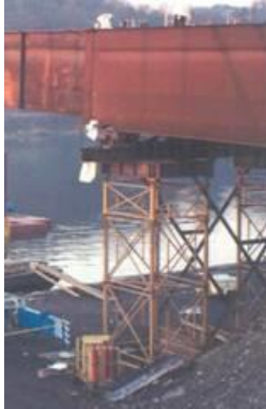
Figure 7 Photograph of a temporary bent
