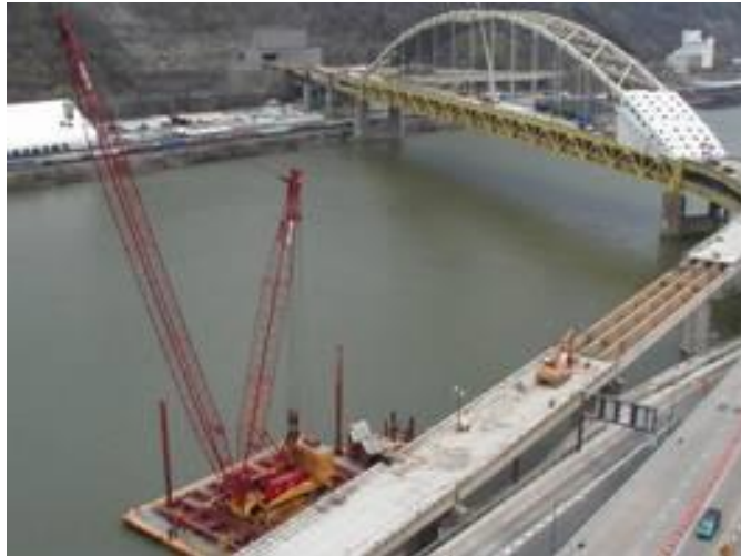
Figure 4 Photograph of a lattice ringer crane
