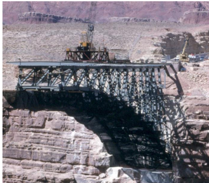
Figure 16 Photograph of an arch bridge erection using the floor system as an erection tie to the canyon wall
