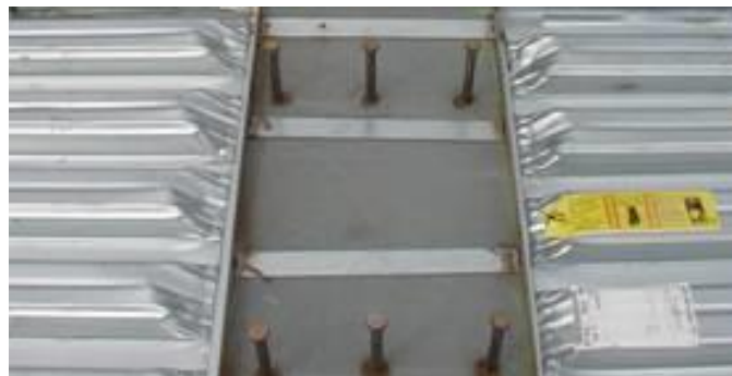
Figure 19 Photograph showing SIP forms attached to a top flange in a tension region
