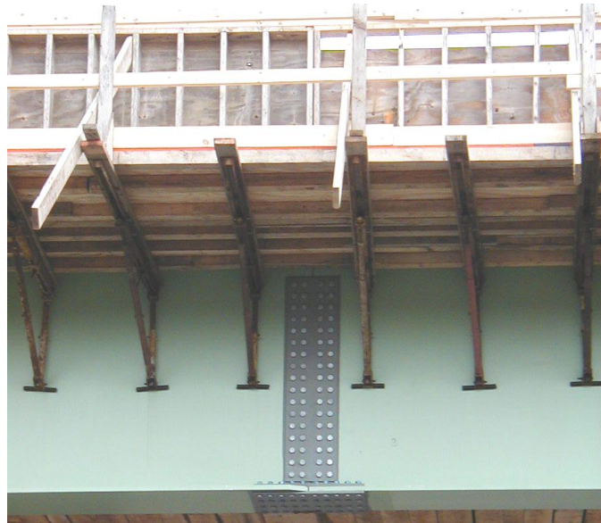
Figure 20 Photograph of a typical overhang bracket
