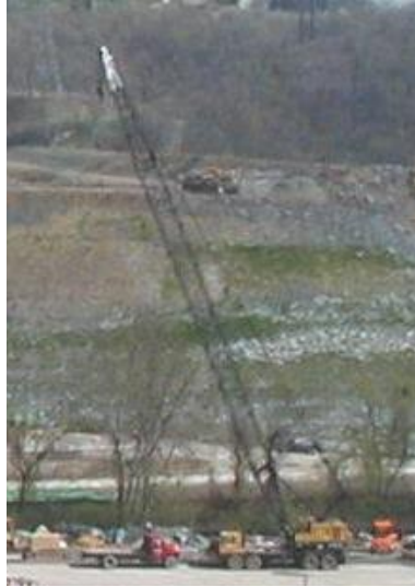
Figure 2 Photograph of a mobile lattice boom crane
