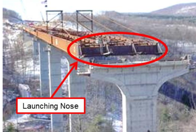
Figure 12 Photograph showing an I-girder launch with launching nose and cable tie-backs
