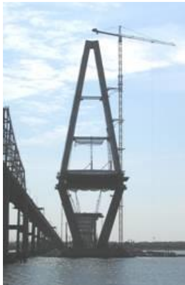
Figure 5 Photograph of a tower crane
