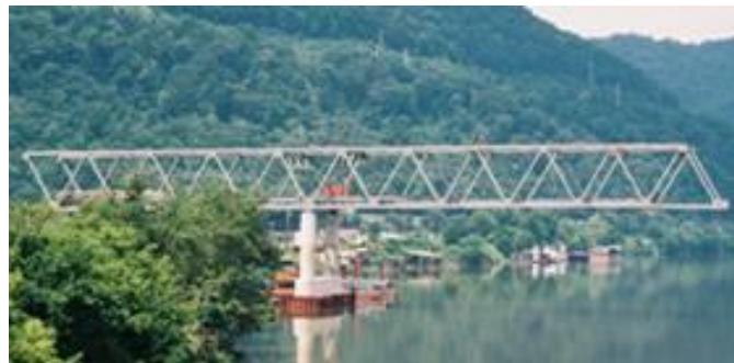
Figure 13 Photograph showing cantilever erection of a continuous truss using barge mounted cranes
